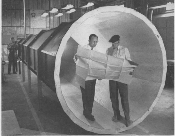
WIND TEST CHAMBER fabricated by the Packaging Division 2232 will be used to test and calibrate instruments for wind, dust and cloud measurements in the Coyote Canyon Test Field. Warren Roberts (5112-2), designer, right, and G. M. Austin (2232-5)
